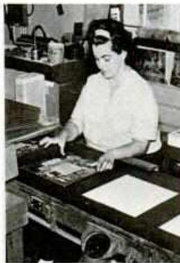
ADVANCE PAPER CO. worker mounts the four-color front on a jacket shell to form an LP container.
